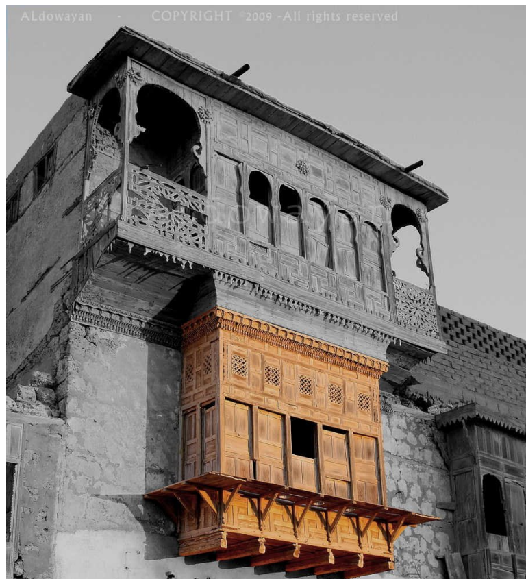
Figure 25. Rawasheen is a type of projected wooden screen in Yanbu Al-Bahr (Source: Photo by Adel Al-Dawayan, Panoramio, 2009)
